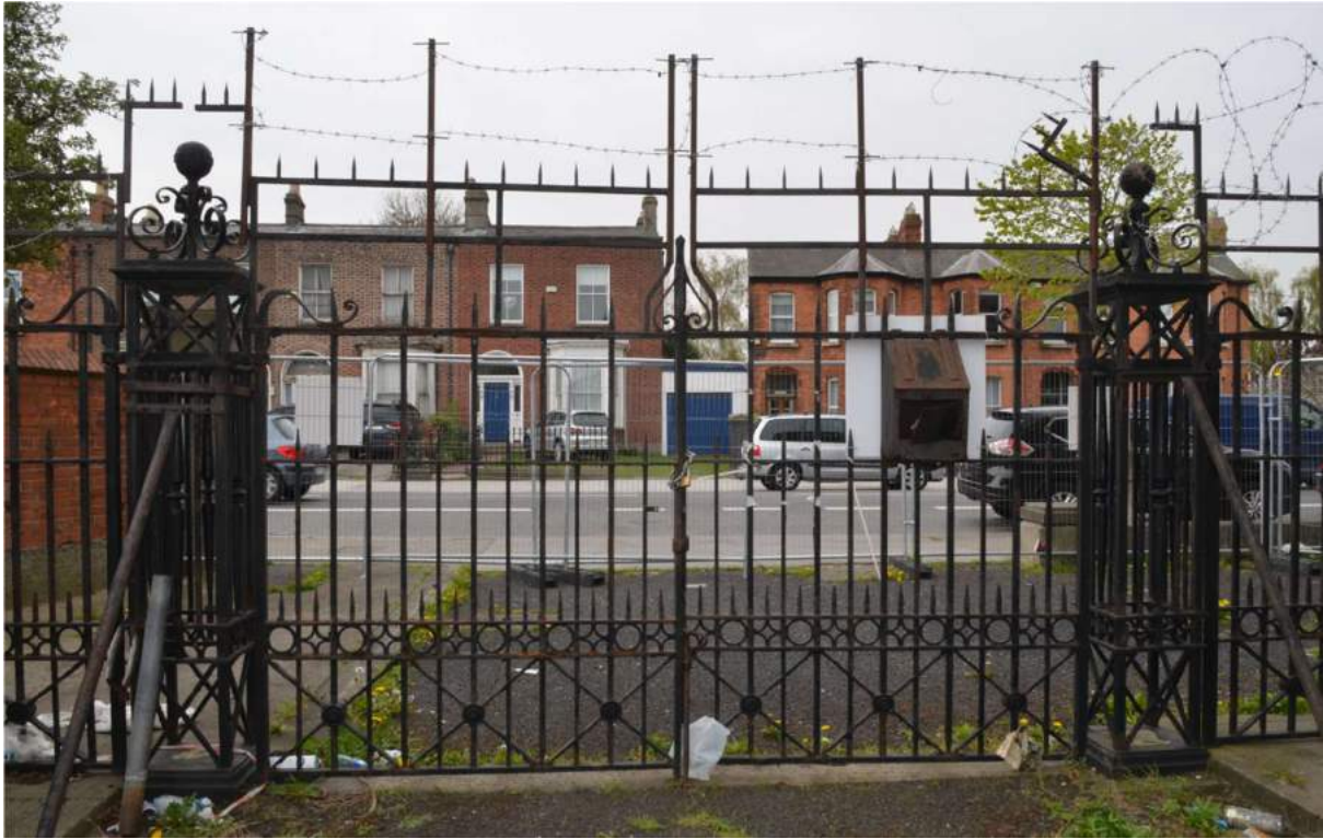
Figure 8: Wrought-iron gates and gate-posts to the South Circular Road.
