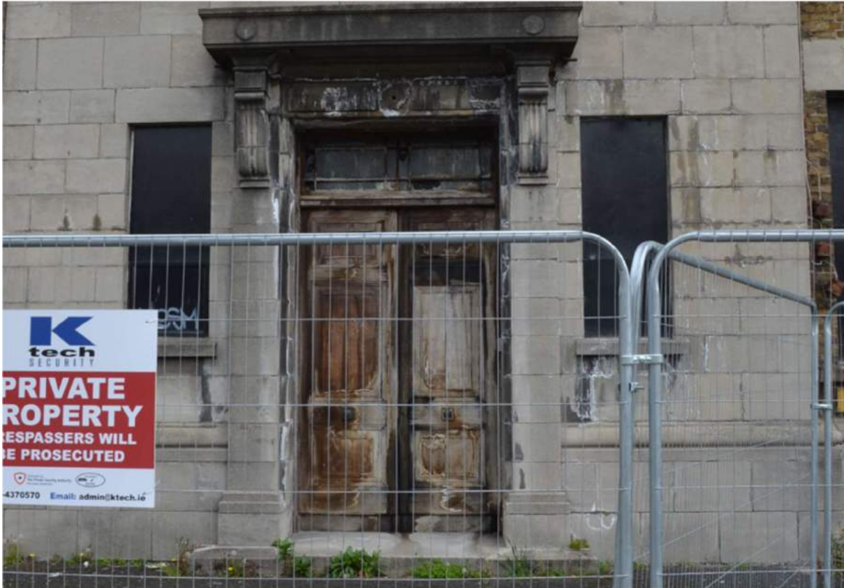
Figure 2: Front entrance door to Factory No. 2 from South Circular Road
