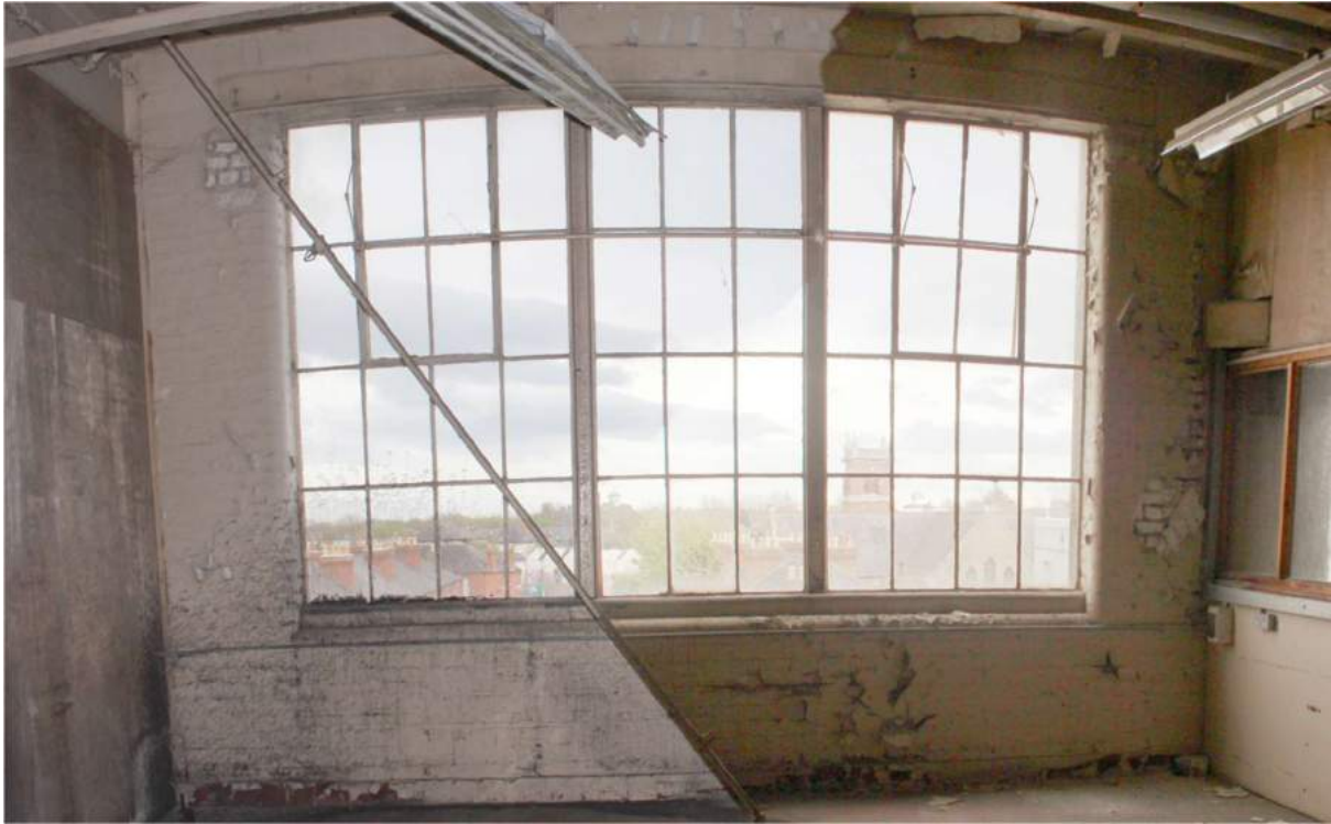
Figure 6: Original steel multi-pane window.
