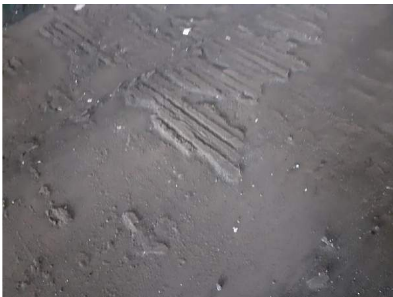
Photograph 2 Undercoat Material First Floor Room
