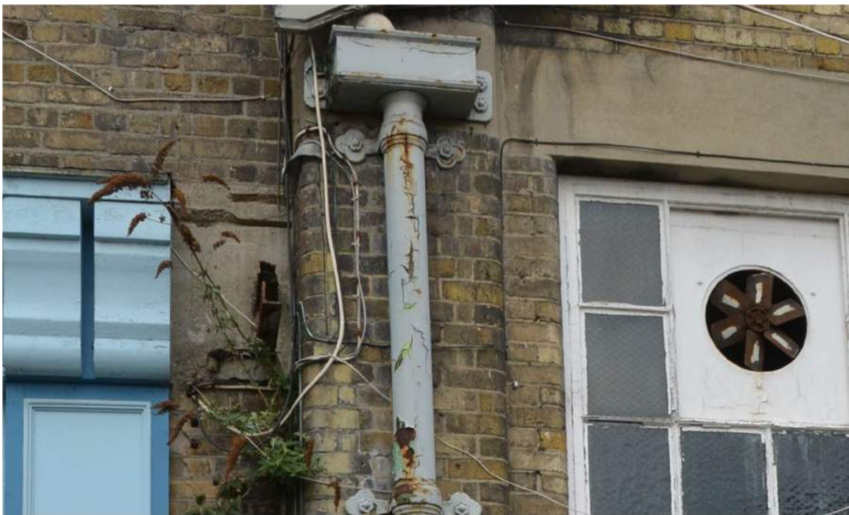
Figure 7: Cast-iron hopper, downpipe and straps.
