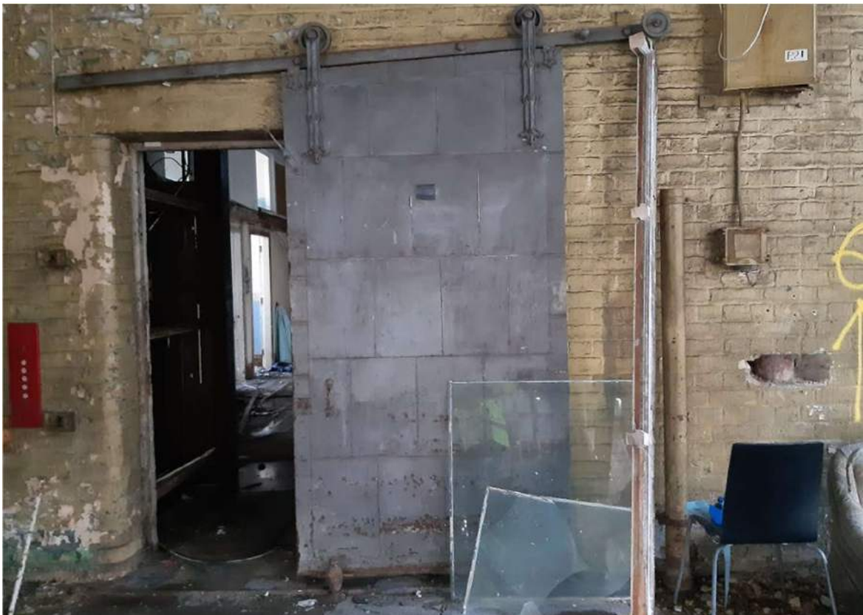
Figure 5: Sliding industrial steel door in Room G.11.
