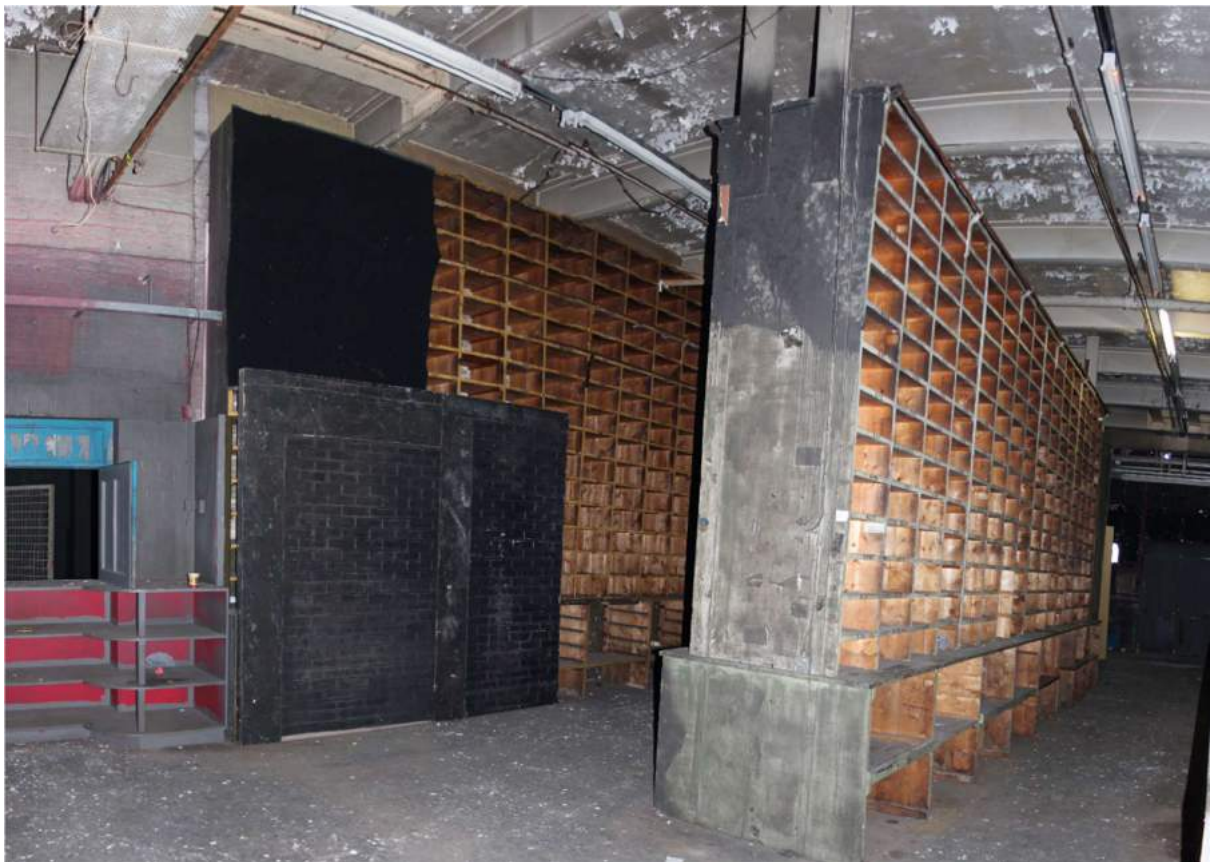
Figure 11: Timber cubby-hole storage in Room G5.
